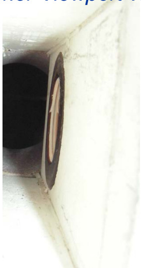
Flow Channel Showing Interior Viewport Window
